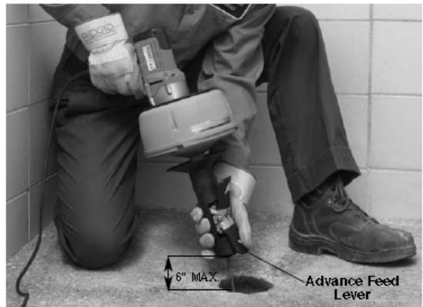
Figure 9 – Feeding Cable With AUTOFEED
